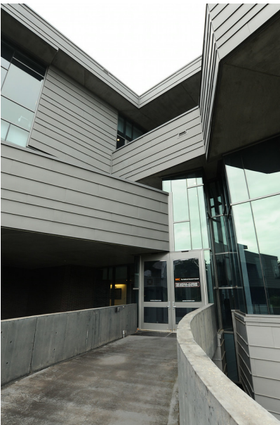
Deep Orange's earliest projects the steel corridors and garages of CU-ICAR's undergraduate engineering center. (Photo/Ross Norton)
